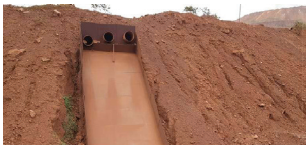
Fig. 5(a). GI sheets with drainage arrangements
