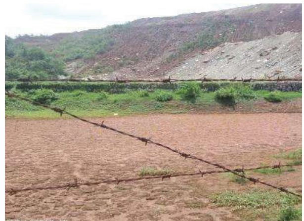
Fig. 4. Settling pit at toe of existing external OB dump with retaining wall
